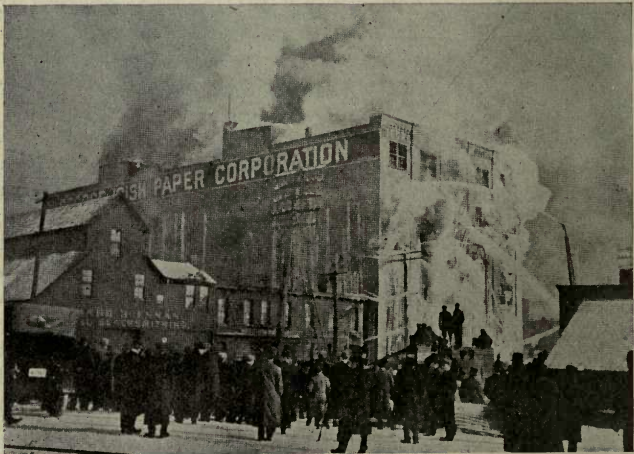
FIG. 3. — Fire in Mill Construction Warehouse of the George Irish Paper Corporation, Buffalo, N. Y.
